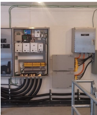
Custom DL Series Dataloggers, Hydro Quebec standards.
